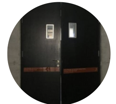
Fire rated escape door
